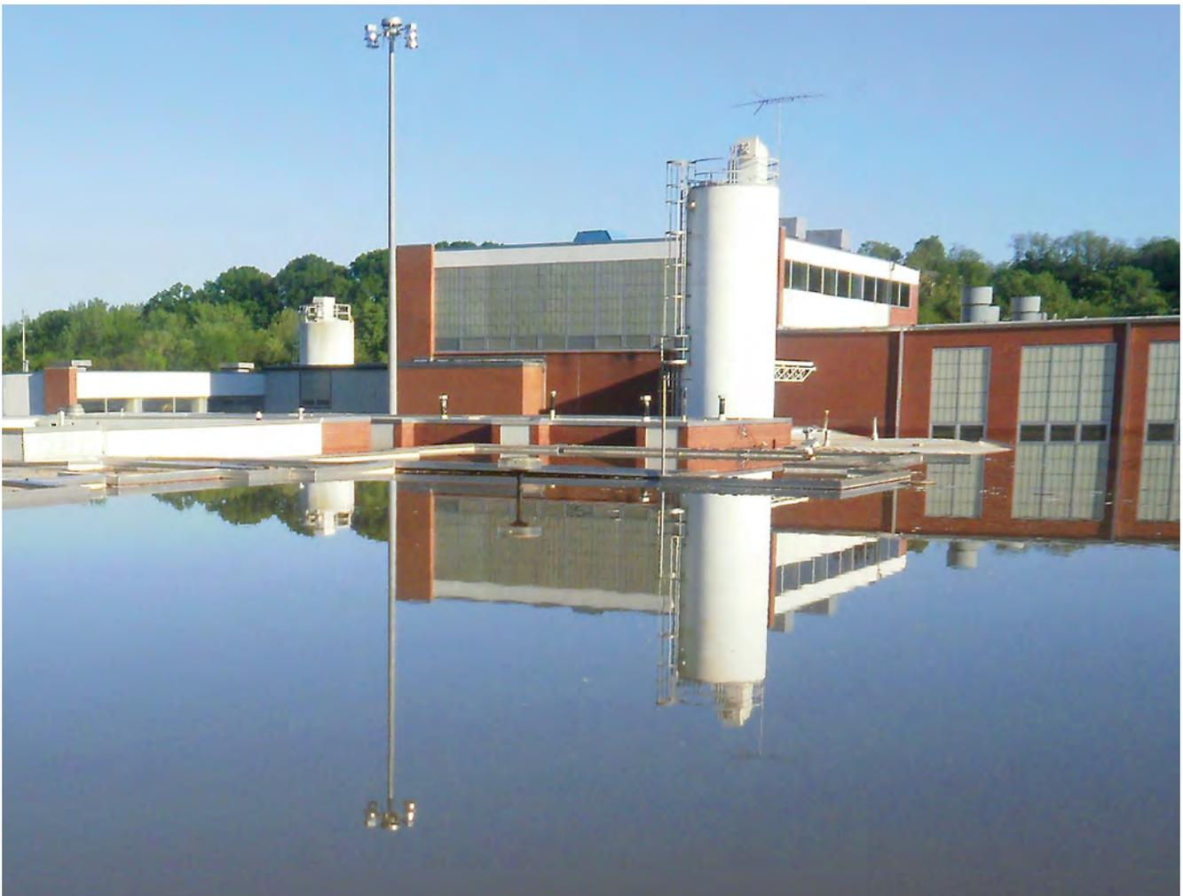
**Clarksville Wastewater Treatment Plant - May 2010:** Levees and floodwalls surrounding the Clarksville WTP were overtopped and the plant was inundated and heavily damaged after the Cumberland Basin received more than 20 inches of rain in less than two days.
