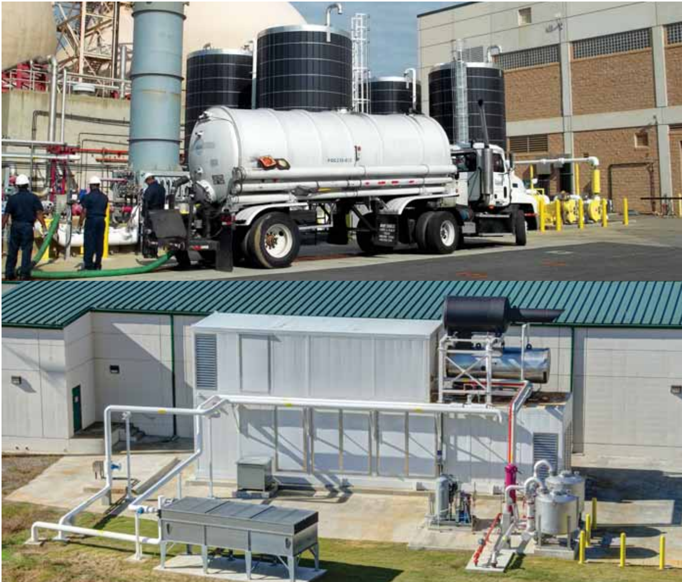
Fats, oils, and grease (FOG) collection at FWHWRC (top photo) provides a robust source of methane gas for the biogas engine generator to convert into electricity (bottom photo), which is used to significantly offset energy costs at the facility.
